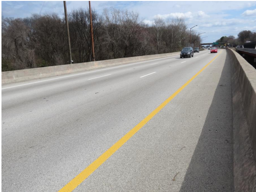
VIEW ACROSS TOP OF WEARING SURFACE WBL
