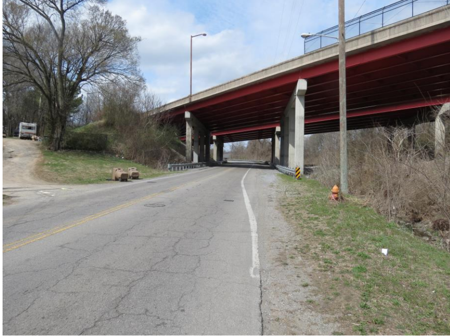
CLEARANCE VIEW RT. SIDE
