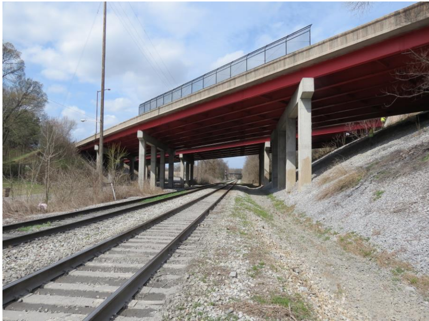
CLEARANCE VIEW RT. SIDE
