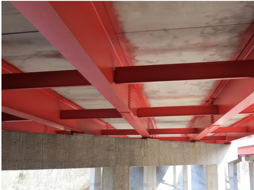
BOTTOM OF DECK VIEW SP. #1
